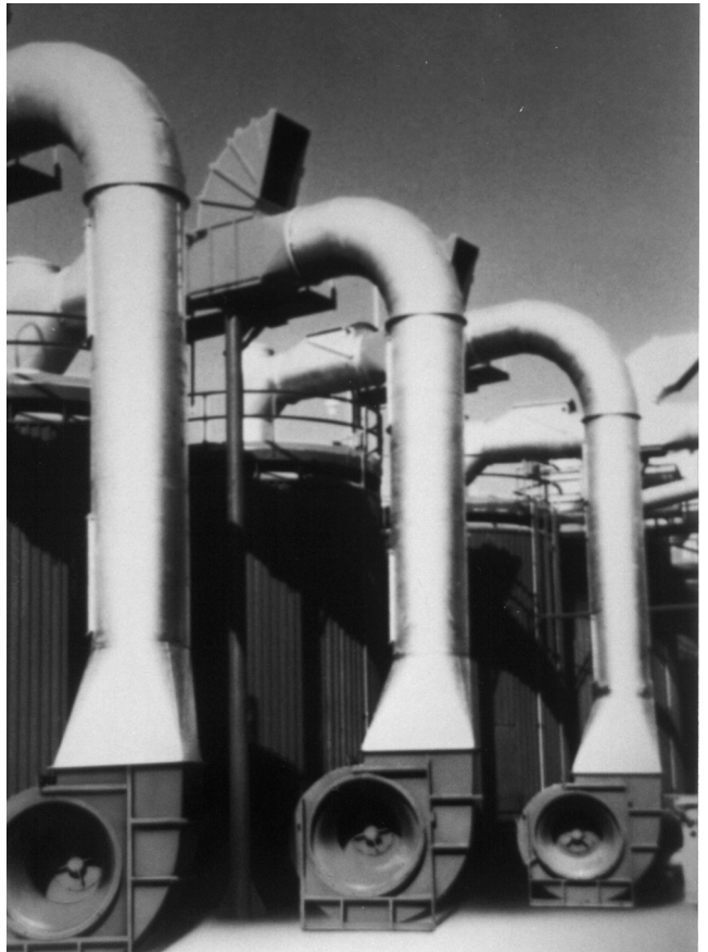
Figure 6. Well-designed duct configuration
