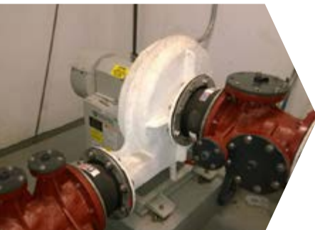
Odor Control Water Treatment
