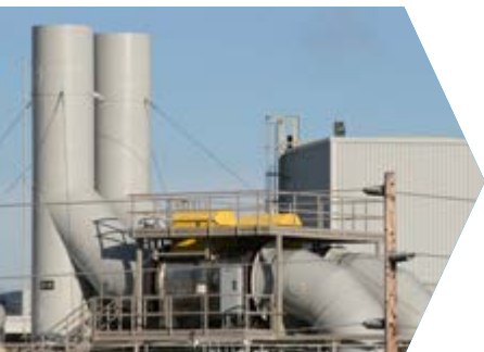
Paint Booth Exhaust
