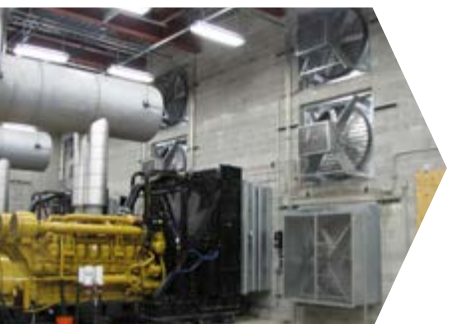
Generator Room Exhaust
