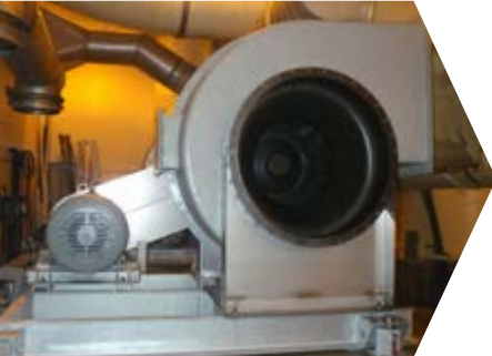
Odor Control Waste Water Treatment
