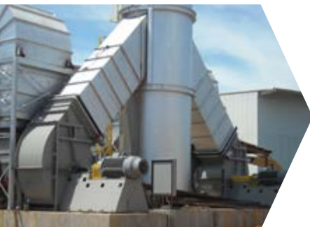
Furnace Room Ventilation
