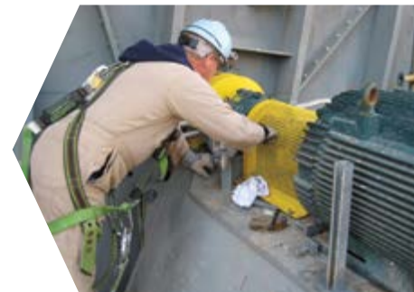
Coupling Alignment
