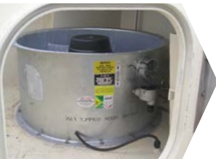
Engine Room Supply Fan (Marine)
