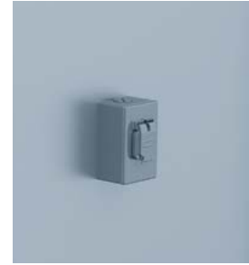
NEMA 3R Disconnect Switch
