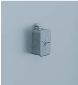
NEMA 1 Disconnect Switch
